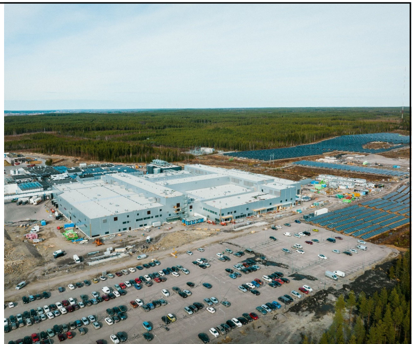
Construction site of the poultry factory in Nurmo, 21 April 2023
